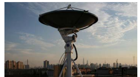
The eOsphere Ground Station installed in Shanghai, China.
